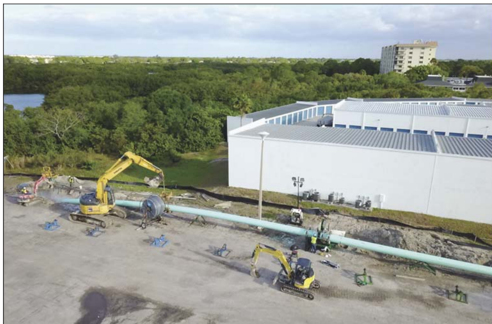
Figure 4. Fusible Polyvinyl Chloride Installation and Fusing Operations
