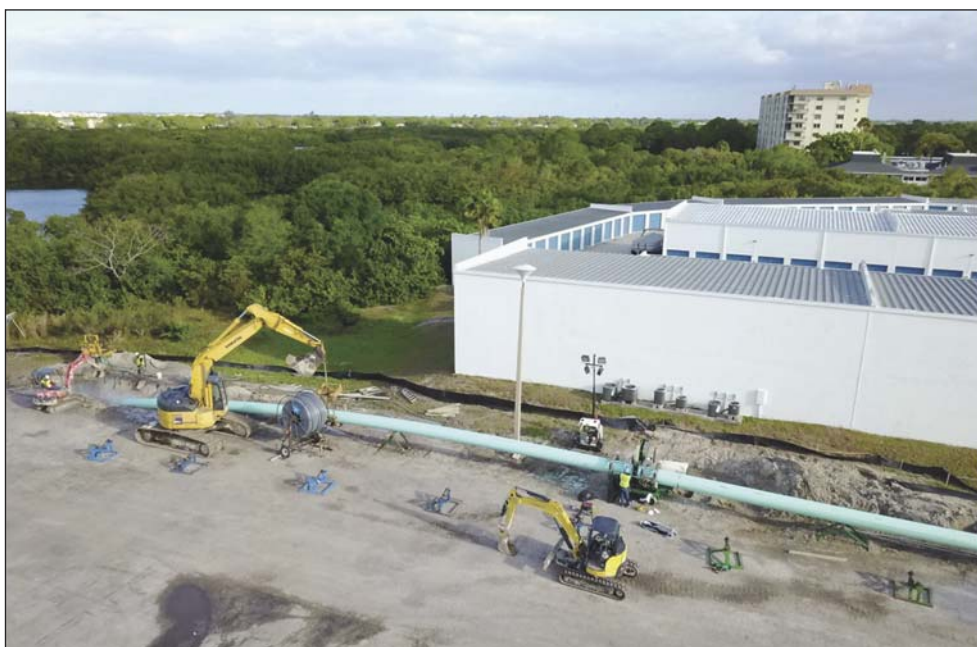
Figure 5. Horizontal Directional Drilling Operations at Park Place Medical Easement
